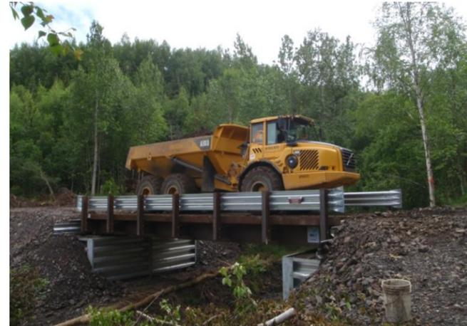
**Temporary bridge and access road:** The Marsh Creek workers built a temporary bridge over Red Devil Creek and roughly a quarter mile of unimproved access road during the 2010 field season. The workers needed the bridge and road to allow heavy equipment to cross the creek without disturbing the creek bed. The bridge will remain until all the cleanup actions are complete and will either be dismantled at that time or left in place at the request of the future landowner.
